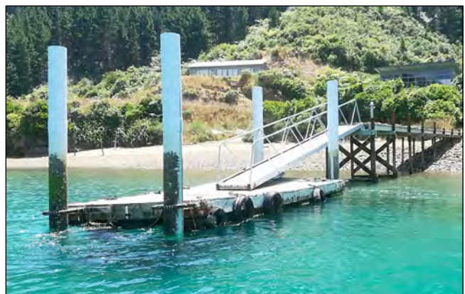
Example of pontoon and pile jetty.
