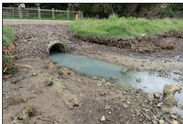
Localised freshwater input from an under-road culvert
