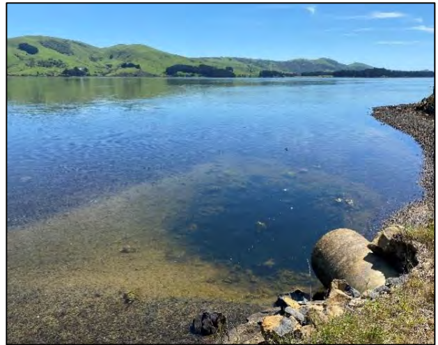
Low oxygen sediment directly below drain outlet
