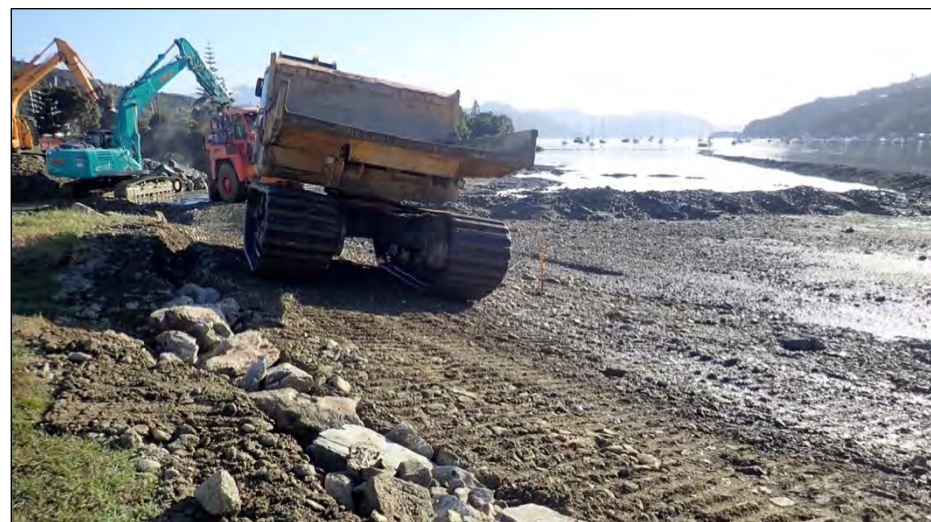
Sediment augmentation requires the use of excavators and trucks
