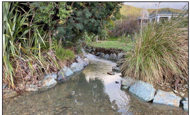
Modified stream entrance with rock placement to minimise erosion
