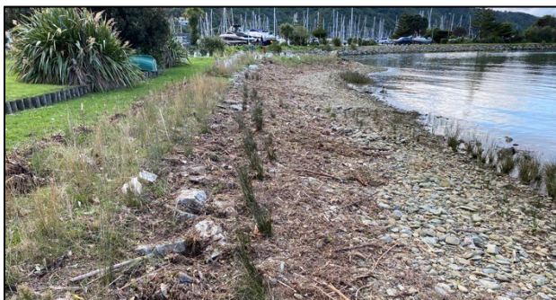
Upper swash zone showing residual organic debris after site clearance. The dark green rushes in the middle of the picture were all buried, but quickly recovered once cleared
