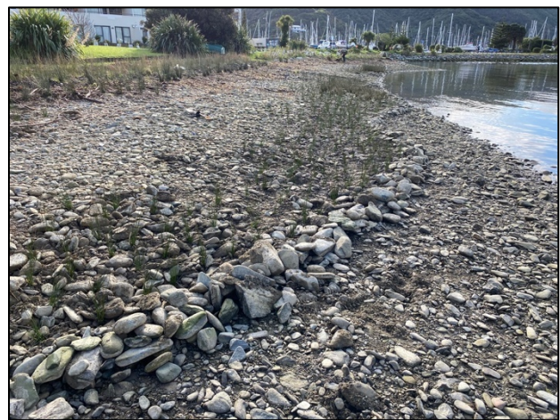
Chenier rock sill seaward of freshly planted searush
